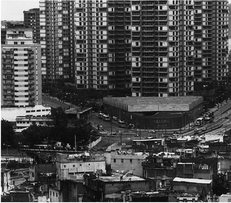
Plate 1.2 Growing cities in less developed nations often have a mixture of modern and sub-standard housing
